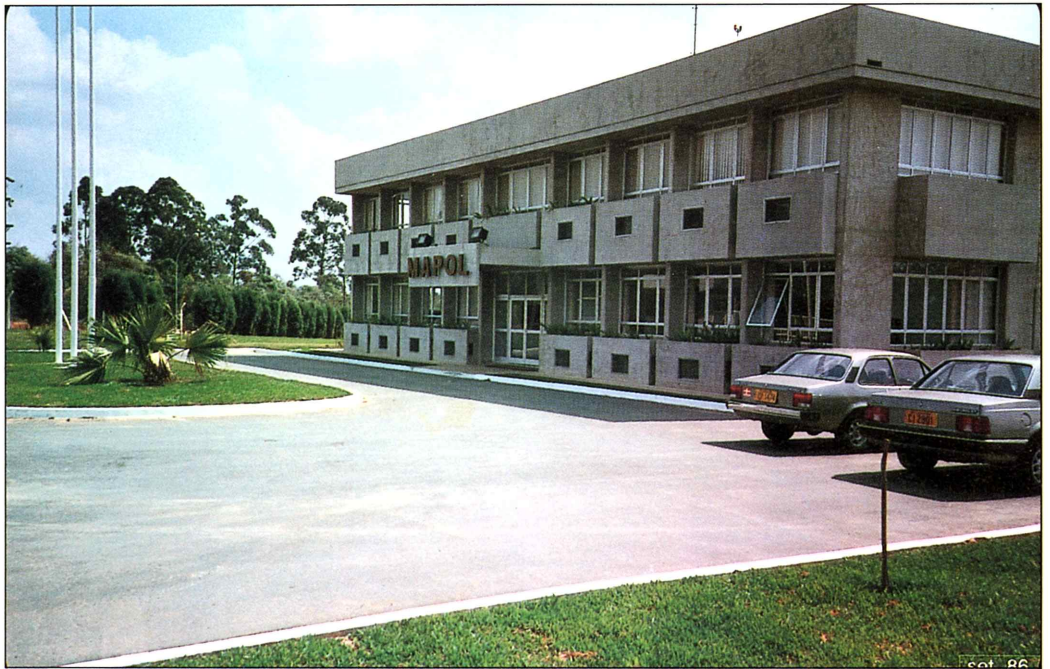
The new office building.
