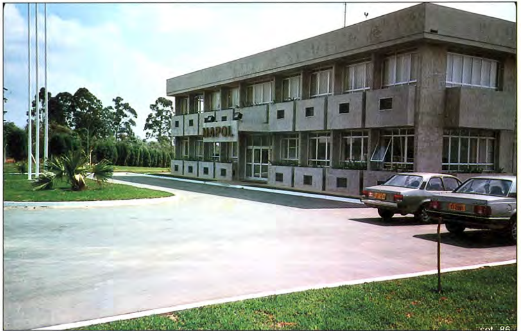
The new office building.
