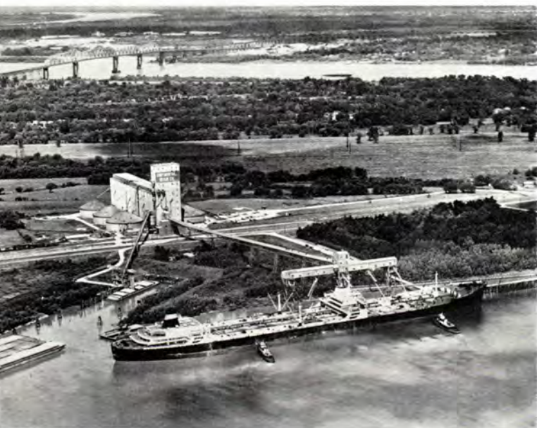
M/S " Manhattan ", large American tanker with a capacity of 108,000 tons grain, loading at Continental Grain's New Orleans, Louisiana, U.S.A. Export Elevator.
