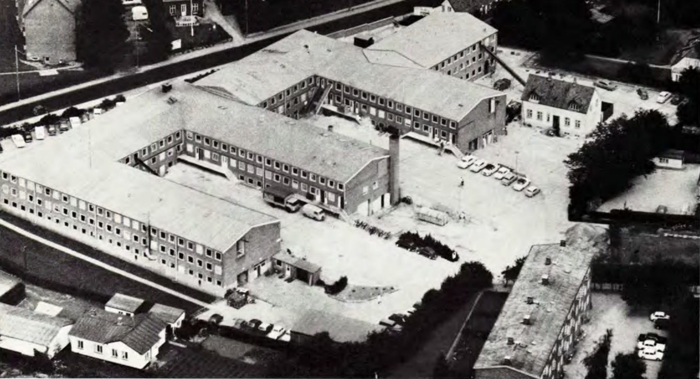
Medicinalcos fabriksanlæg i Nærum. The industrial plant of Medicinalco Ltd. at Nærum, just outside Copenhagen.
