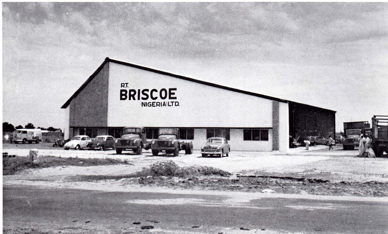
The new workshop at Kano, Northern Nigeria.
