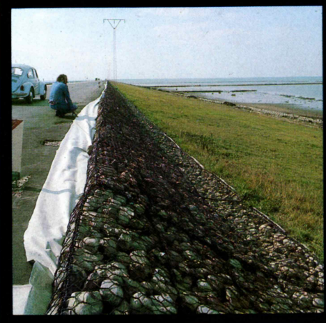
Faserne i sikringen af Rømø-dæmningens sider. Stages in connection with safeguarding the slopes of the Rømø causeway.
