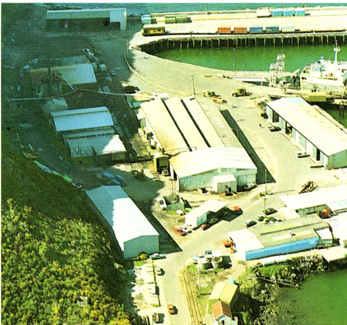
Dry mill installations at the Port of Stanley.
