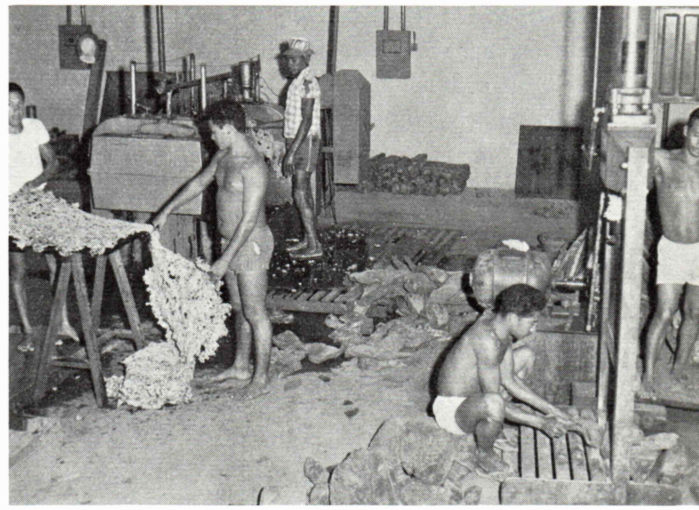
Brasilien. Gummikuglerne skæres op, før de går i vaskemaskinen. Bagefter bliver de valset til »sheets«. Brazil. The rubber balls are cut to pieces before they are put into the washing machines. Afterwards they are milled into sheets.
