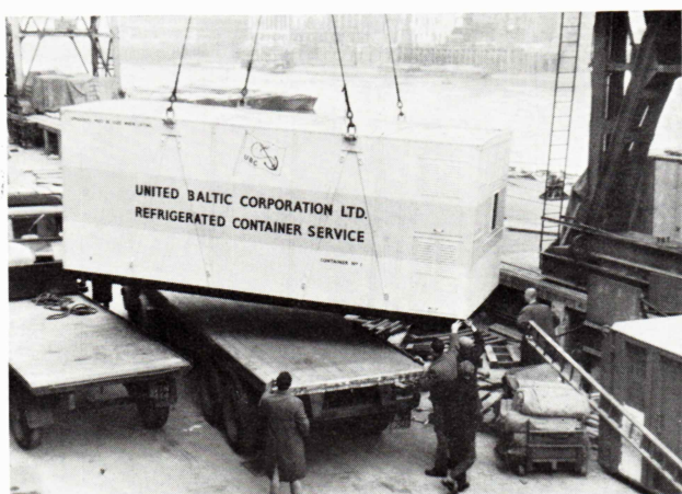
London. From the lorry the container is lifted by a crane and placed directly on board the ship.
