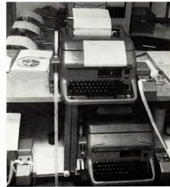
Copenhagen. The transmitting equipment in the TEXCOM-circuit Copenhagen - Hong Kong. All transmitting is being done by means of code tapes. Underneath a perforating machine making the code tapes.
