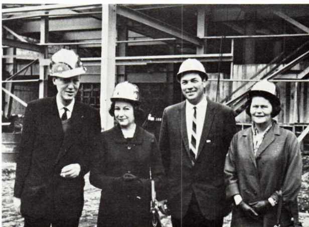
Gold River. Princess Anne, Prince Georg, Mr. Bruce Chisholm (Reeve of Gold River Municipality) and Mrs. J. Vibe Christensen in front of the steel framework of the new power house, Gold River pulp mill.
