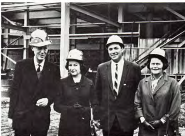
Gold River. Princess Anne, Prince Georg, Mr. Bruce Chisholm (Reeve of Gold River Municipality) and Mrs. J. Vibe Christensen in front of the steel framework of the new power house, Gold River pulp mill.
