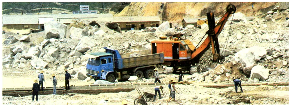
Excavation is done by modern excavators, heavy-duty lorries, as well as primitive carts provided with strong bicycle wheels.
