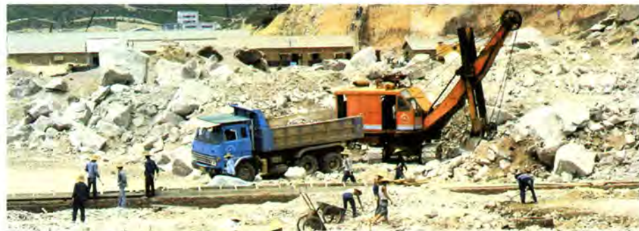
Excavation is done by modern excavators, heavy-duty lorries, as well as primitive carts provided with strong bicycle wheels.
