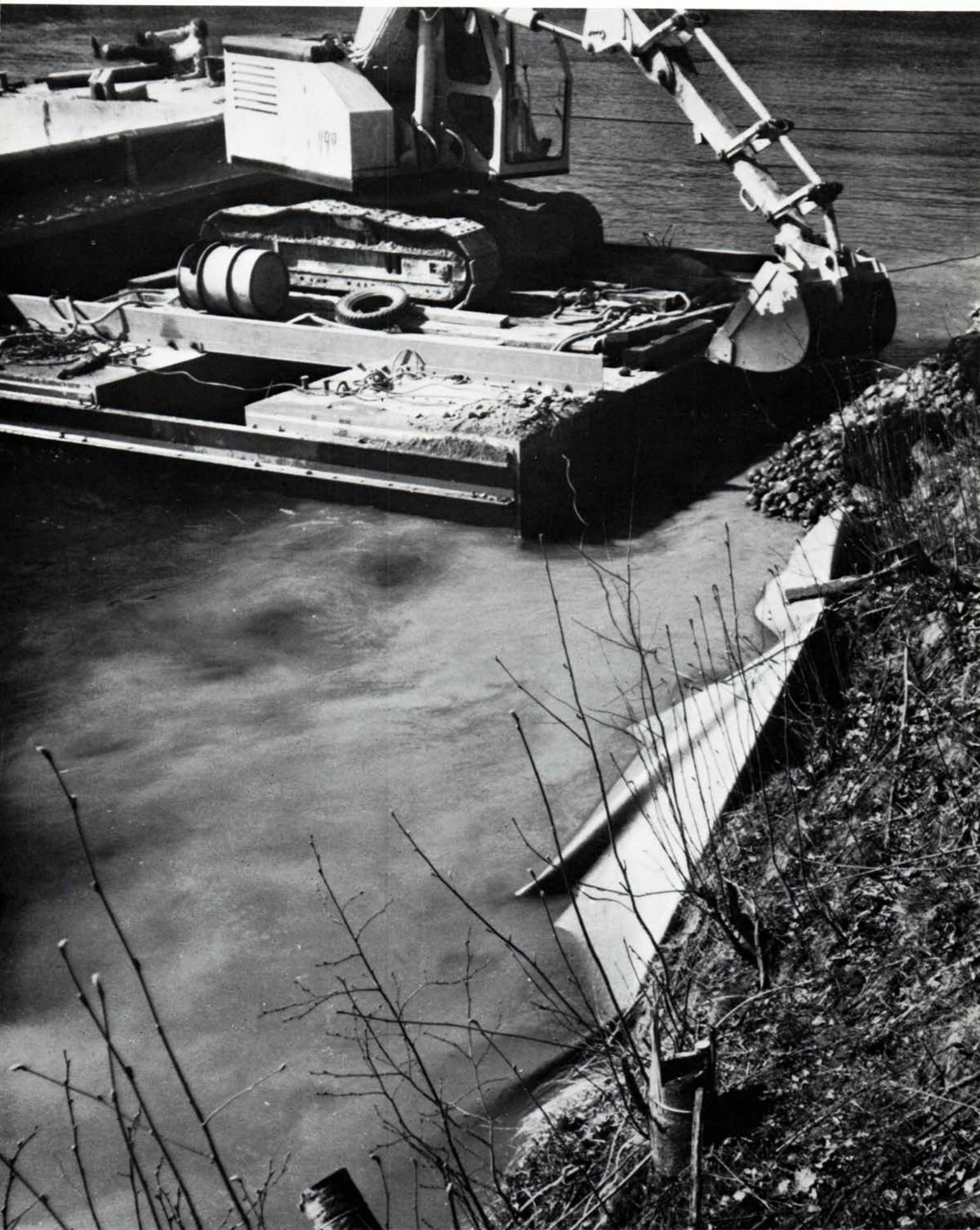
Fibertex som erosionsbeskyttelse af flodbred. Fibertex used as protection against erosion of river banks.
