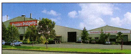
The wool-washing facility in Auckland.
