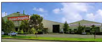
The wool-washing facility in Auckland.
