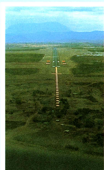
Chileka-lufthavnen i Malawi med landingslyset for fuldt blus. Chileka International Airport in Malawi with the landing lights switched on at full capacity.
