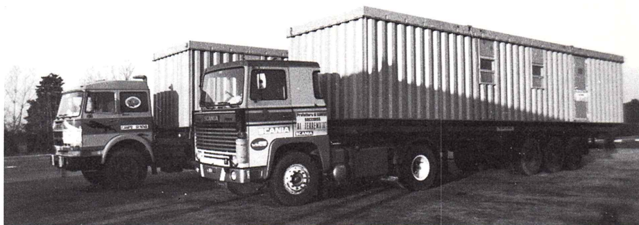
The two prefabricated houses ready to leave Genoa.
