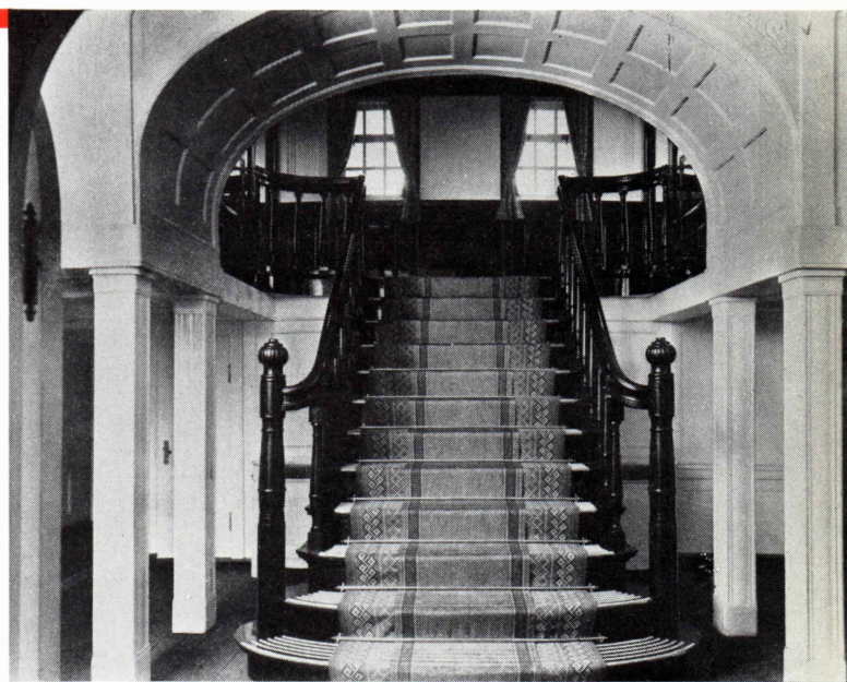
Trappen op til rygesalonen. The staircase leading to the smoking saloon.
