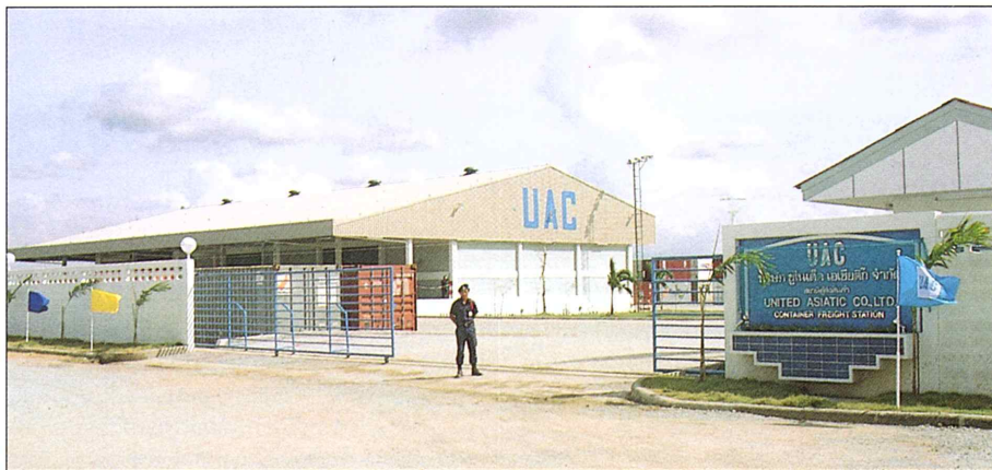
The new container terminal has a 24-hour guard
