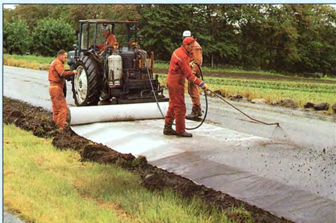
Fibertex products are used for the renewal of road surfaces and other purposes.
