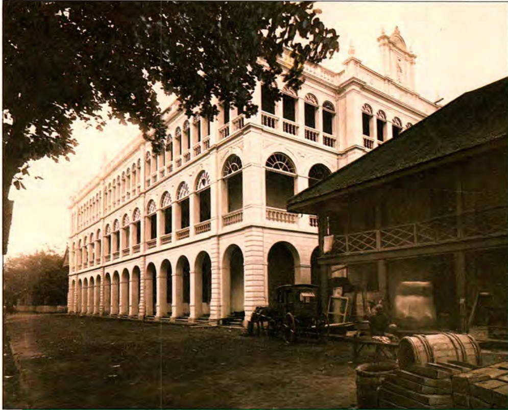
The Bangkok office under construction. In the foreground, the original Andersen & Co. building
