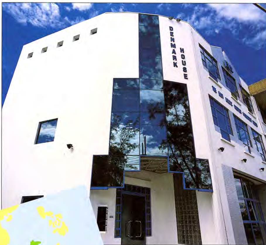
Denmark House, EAC's new office building in Kota Kinabalu
