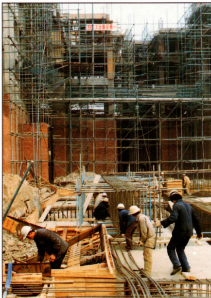
Workers are busy on the project.
